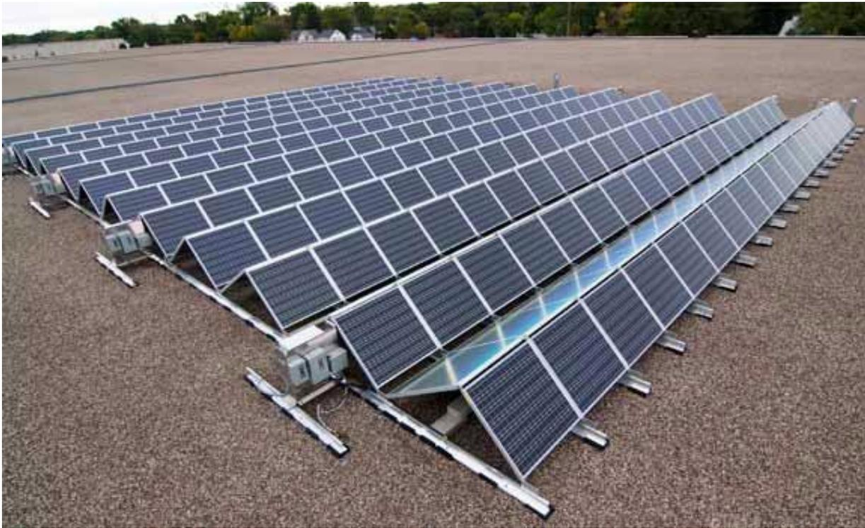
**Shade** tolerant designs can be attractive when space is constrained or, when output can be enhanced, as in this case using mirrors; ***System-level advantage***
