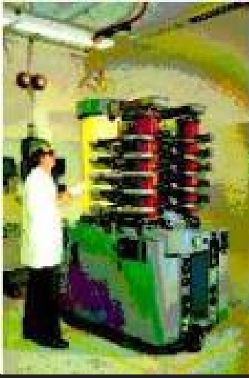
Mercury Arc Valve HVDC (Phased out)
